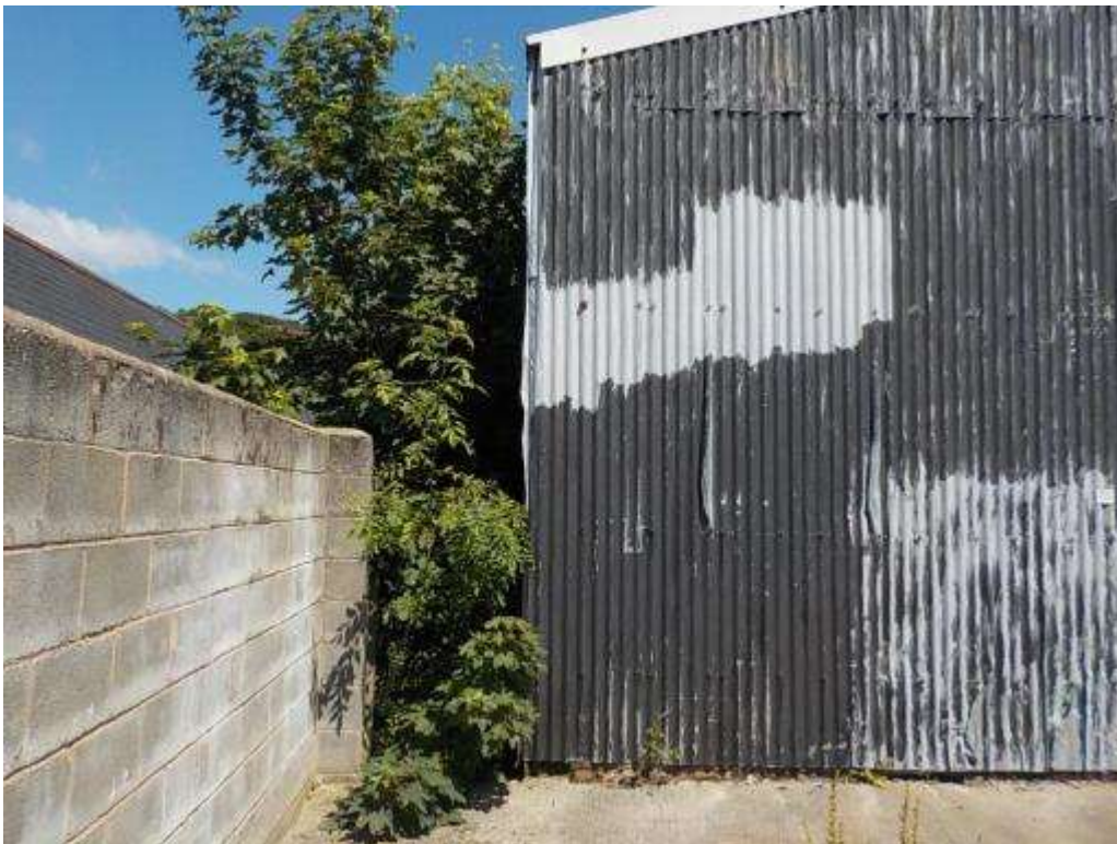
Small areas of scrub between sides of the shed and the site boundary wall
