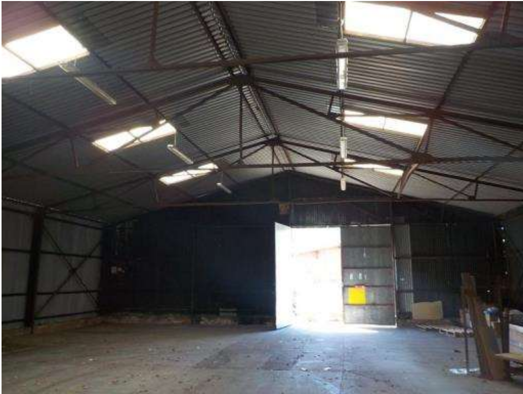
Interior of the shed
