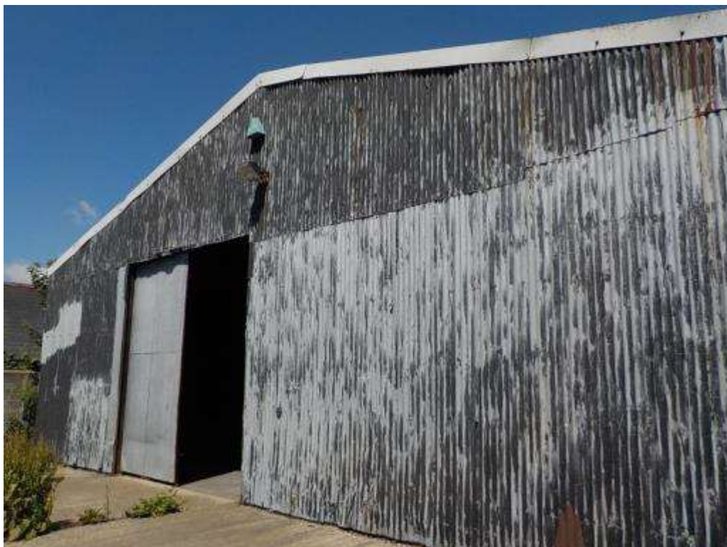
Rear elevation of the shed
