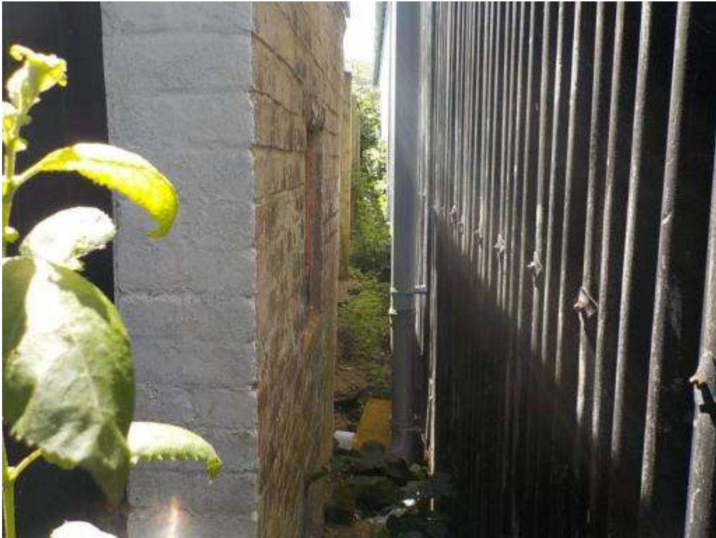
Edge of the small toilet block and shed wall
